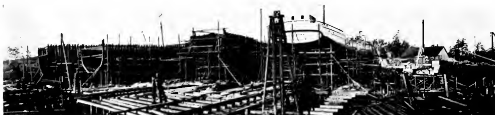
General view of the Cameron-Genoa Shipbuilders, Ltd., plant at Victoria, showing work under way.
